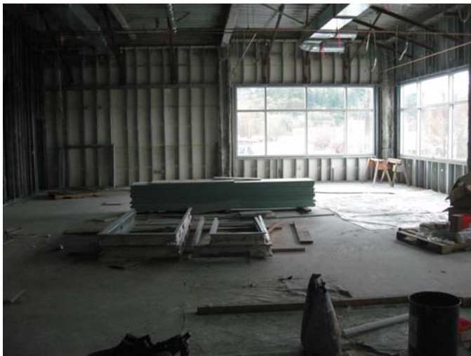
2nd floor—community meeting room, southeast corner
