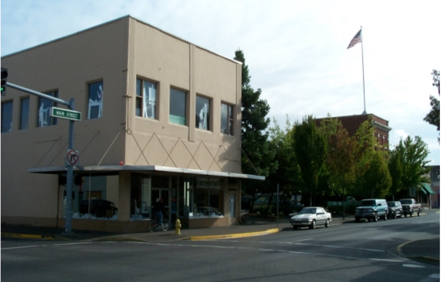
The Gerlach building on Springfield's Main Street.
