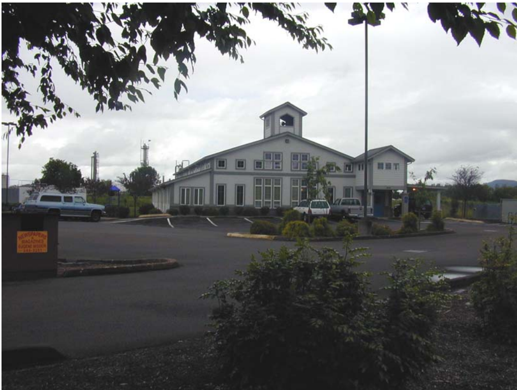
Goodwill Day Care West Side of 30 th Street
