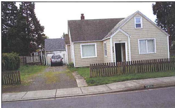
Existing dwelling fronting West M Street
