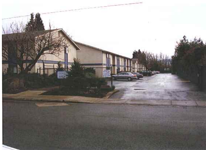
Centennial Apartments – Located east of Rainbow Drive
