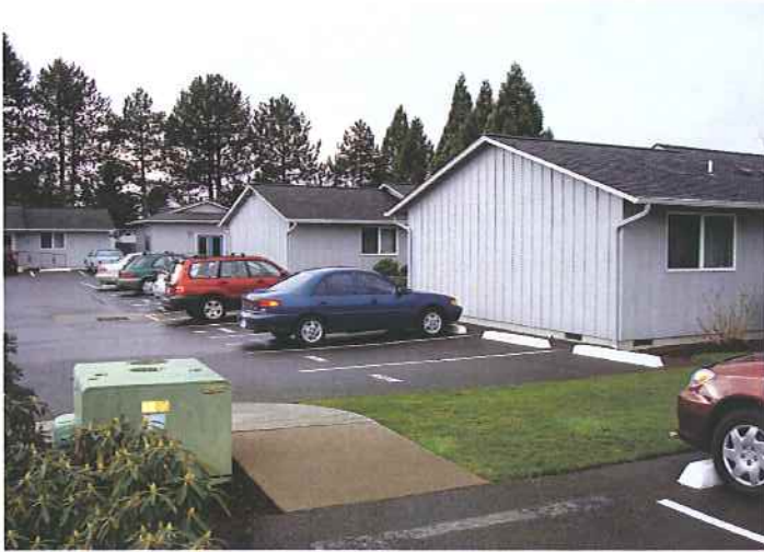
Biccennial Condominiums – Stage 2 Approximately 17 Dwelling Units per/acre Located west of Rainbow Drive
