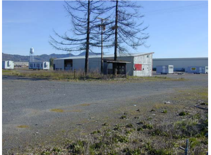
Existing empty structures on TL 400
