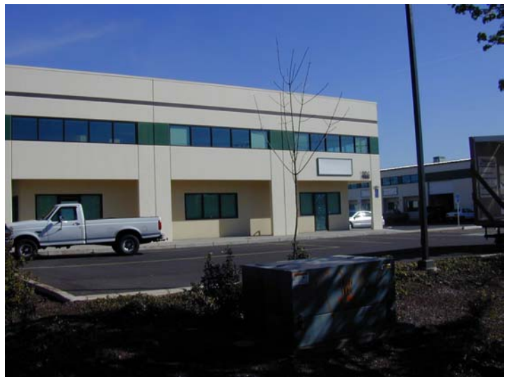
Existing business park on property located east of TL 400
