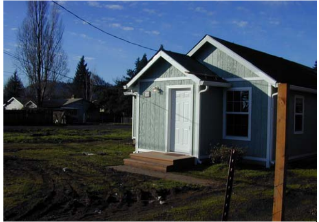
Neighboring single family home located on lot to the north
