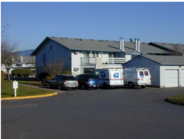
Medium Density development (apartment complex) located across the street from proposed rezone.
