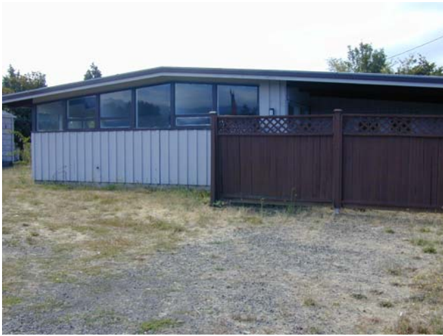
Existing structure on site.
