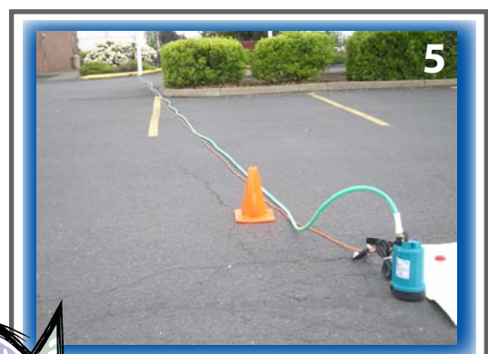
Step 3. Place the pump on the low side of the drain cover where the water will collect. Once water starts to pool check to be sure the pump is in the water. Attach garden hose to pump (at black adapter location). A “snug” fit will do...forcing it more than this may strip the adapter and cause it to leak. NOTE: Attach the end with the swivel for easier turning.
