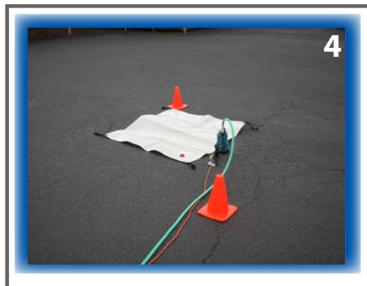
Step 4. Place a cone on both sides of the drain cover.
