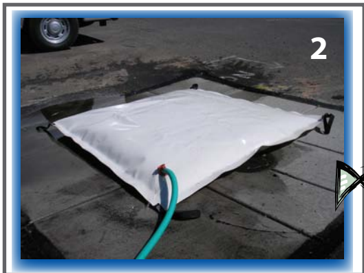
Step 2. Use garden hose to fill white drain cover to form a seal over the drain.
